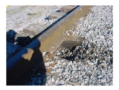
This photo shows a properly prepared crib providing the room required to bolt the sensor-mounting bracket to the rail.
