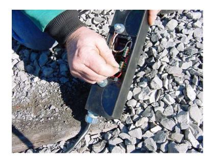
This photo shows the installer pushing the wire into the spring cage connector. Always tug on the wire, after pushing the wire into the connector, to assure a good "bite" of the spring cage on the wire.
