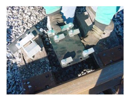
It is necessary to rotate the clamp hooks so that they are parallel with the rail. This provides the clearance required to place the baseplate firmly in contact with the underside of the rail. The bolts on the clamp hooks should
