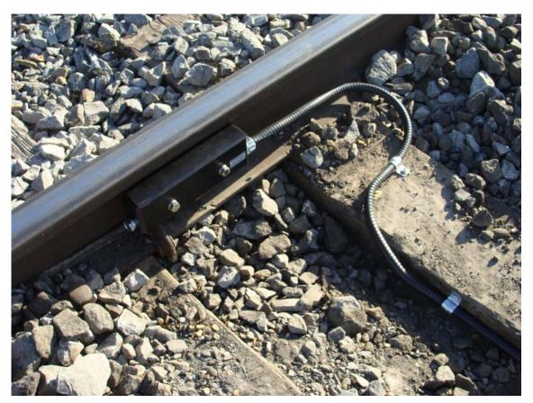
As shown in the above photo, leave enough extra cable so as to allow movement of the rail and re-wiring of wheel sensors in future.
