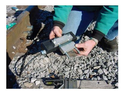
It is now time to select the appropriate spacers to provide the correct mounting height of the wheel sensor relative to the top of the rail. The correct distance to set the top of the wheel sensor from the top of the rail is 1-3/4" (+1/16" or -1/16"). The larger the rail size the more spacers are required to accomplished this.
