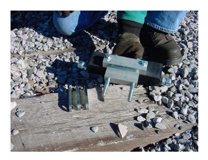
Remove the spacers and the mounting bar from the wheel sensor.
