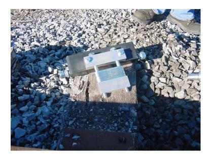
The sensor head assembly includes the wheel sensor, the spacer kit, mounting bar and associated bolts, washers and nylock nuts. Removal of this assembly is necessary to allow the installer to attach the baseplate to the underside of the rail.
