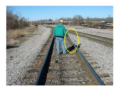
This photo shows the correct "right side" orientation of the sensor when facing the switch. The installation of the sensor on the right side is true regardless of whether the installer is facing the switch from the facing or trailing side of the points.
