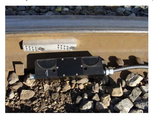
When the proper threaded holes have been determined the wheel sensor can be final tightened to the rail mount adapter.
