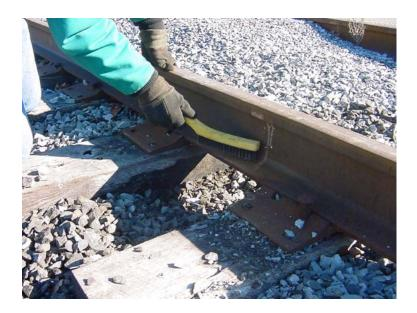
It is necessary to clean the rail to assure a secure connection between the mounting bracket and the rail. A wire brush should be used to clean foreign material from the top, sides and underside of the rail at the location the mounting bracket is to be attached.
