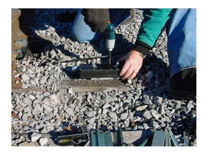
Wiring the Wheel Sensors: Attach communication cable wires to the sensor head. This should be done prior to attaching the sensor to the bracket assembly. Run the (# 18 – 4 conductor) communication cable beneath the rail in the crib space area that was previously cleaned out. Remove the black aluminum cover on the backside of the wheel sensor.
