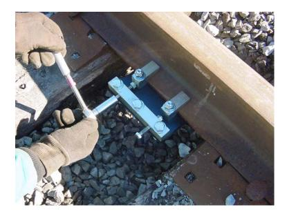
Begin tightening the take-up bolts located on the thrust bar on the field side of the baseplate. This action will snug the clamp hooks up against the sides of the base of the rail.
