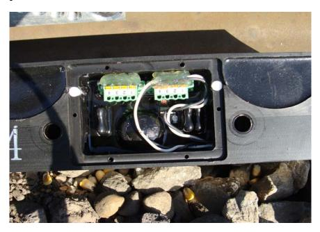
The wheel sensor can now be bolted to the rail mount adapter. Using a combination square with a bubble level, determine which threaded hole sets will place the wheel sensor at the 1-3/4" recommended height.
