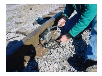
Note: Do not make direct vertical cable runs to the Wheel Sensors. Always allow extra cable to accommodate track heaving and future Wheel Sensor replacement.
