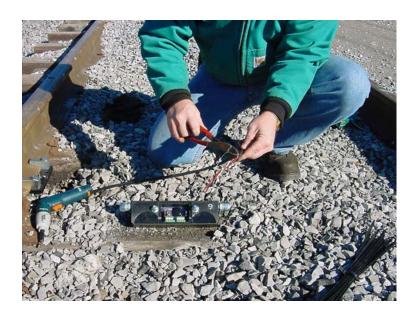
Insert the stripped wire through the cord grip on the end of the wheel sensor. Insert the wires into the spring cage connector by pushing the stripped wire ends into the appropriate terminals.
