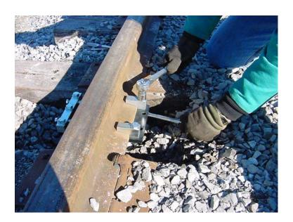
Securely tighten the bolts that hold the clamp hooks to the baseplate. Be sure to tighten all (4) clamp hook bolts evenly.
