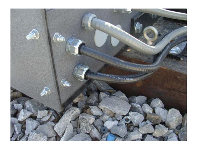
The photo above shows two separate sensor cables entering the Switch Machine. One of the cables would be routed to the facing point wheel sensor/sensors. The other sensor cable would be routed to the trailing point wheel sensor/sensors.
