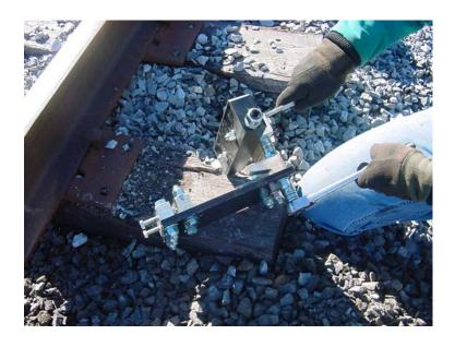
Remove the sensor assembly from the mounting bracket rail plate.
