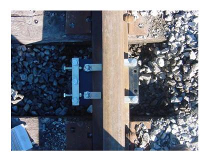
The clamp hooks should be rotated so that they extend over the base of the rail. It may be necessary to loosen the clamp hooks slightly on larger rail sizes in order to allow for the clearance needed to rotate the clamp
