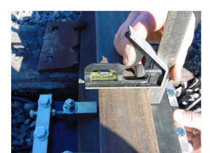
After determining the correct number of spacers required for the installation of the wheel sensor, it is necessary to place the unused spacers beneath the baseplate. The spacers located on the bottom are required to assure that the spacer stack is securely tightened before the thread limit is reached on the bolts.
