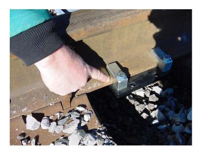
Tighten the take-up bolts until there is no gap between the side of the rail base and the inside of the clamp hooks.
