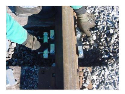
Place the baseplate assembly beneath the rail in the crib space area previously cleared away.
