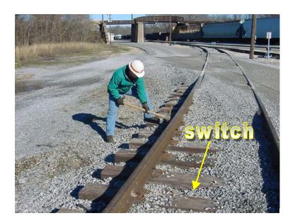
The location of the wheel sensors would have been determined, as previously discussed, based on the track geometry. It is necessary to remove the ballast from the crib space between the ties where the sensormounting bracket is to be installed.
