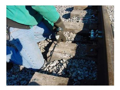
The cable should be either secured to the top of the ties or buried at a location that will allow normal track maintenance to occur without contact of the cable being possible. RTI strongly recommends that the communication cable from the wheel sensors be buried. This is the most secure and trouble free method of installing the cable for long term operation. Attaching the cable to the ties should be used in applications where the wheel sensors are being installed for test or short-term purposes.
