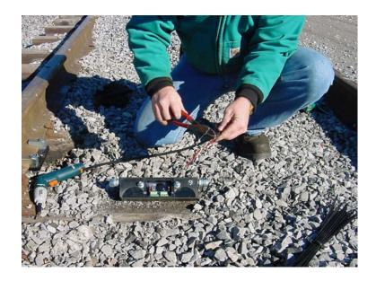
Insert the stripped wire through the cord grip on the end of the wheel sensor. Insert the wires into the spring cage connector by pushing the stripped wire ends into the appropriate terminals.
