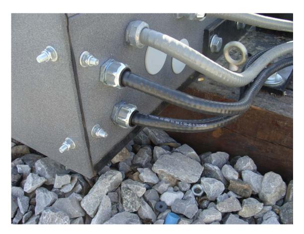
The photo above shows two separate black sensor cables entering the Switch Machine. One of the cables would be routed to the facing point wheel sensor/sensors. The other sensor cable would be routed to the trailing point wheel sensor/sensors.
