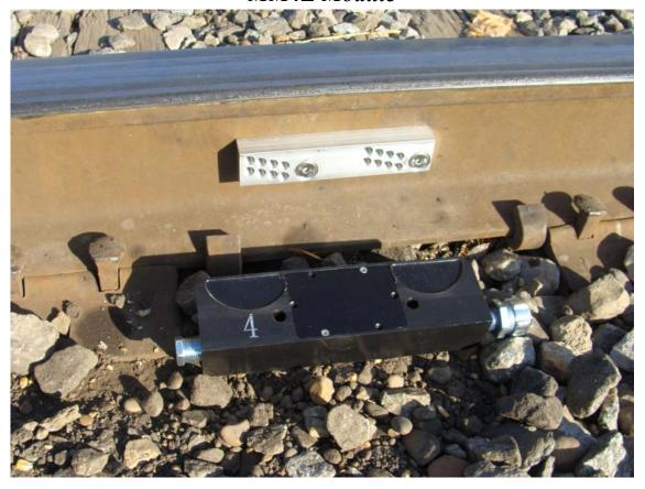
Select the appropriate wheel sensor and bracket assembly for installation at the location prepared to receive the assembly. This photo shows the sensor used at an end of run or for example a single facing point sensor. One end of the sensor has a cord grip to allow the installation of the communication/power cable. The other end has a plug to prevent the entrance of moisture and contaminants into the wheel sensor.
