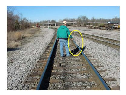
This photo shows the correct "right side" orientation of the sensor when facing the switch. The installation of the sensor on the right side is true regardless of whether the installer is facing the switch from the facing or trailing side of the points.
