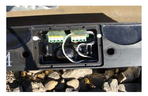
This photo shows a correctly wired wheel sensor that is an "end of run" or facing point location. Notice the oxide inhibitor grease is applied on both connectors even if wires are not in the connector to keep moisture and contaminants from entering the connector.
